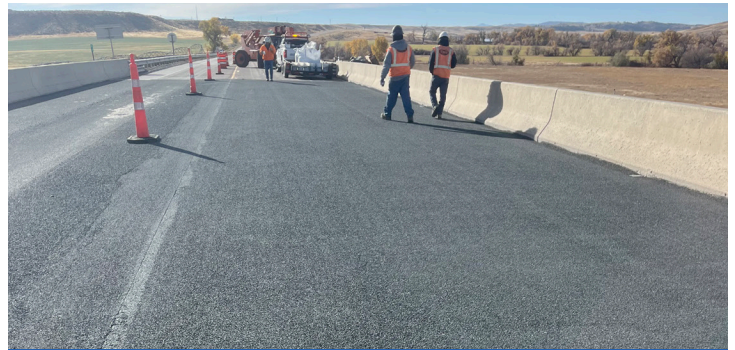
Bridge deck overlay
