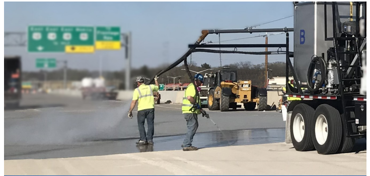
Bridge deck overlay
