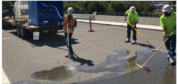
Bridge deck overlay
