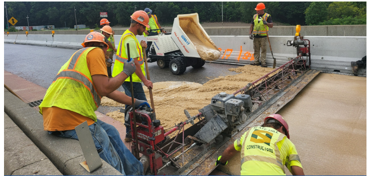
Bridge deck overlay
