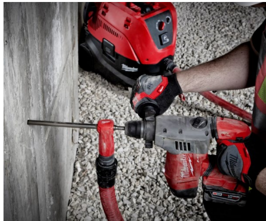
FIGURE 8— MILWAUKEE VACUUM BIT SYSTEM
